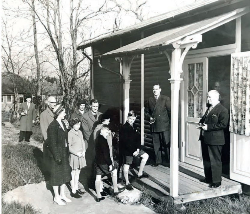
Where it began – Guide Hut Semley Road, temporary
